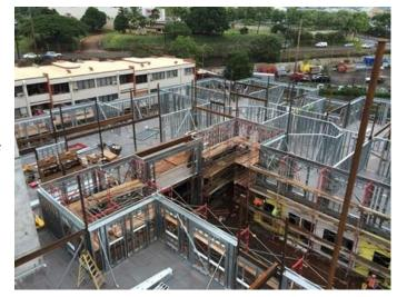
precision in the framed structure. There were concrete shafts that needed to match the settlement with the framed walls along with structural steel members in select areas of the building, putting greater emphasis on panelization consistency. Group Builders chose CEMCO
